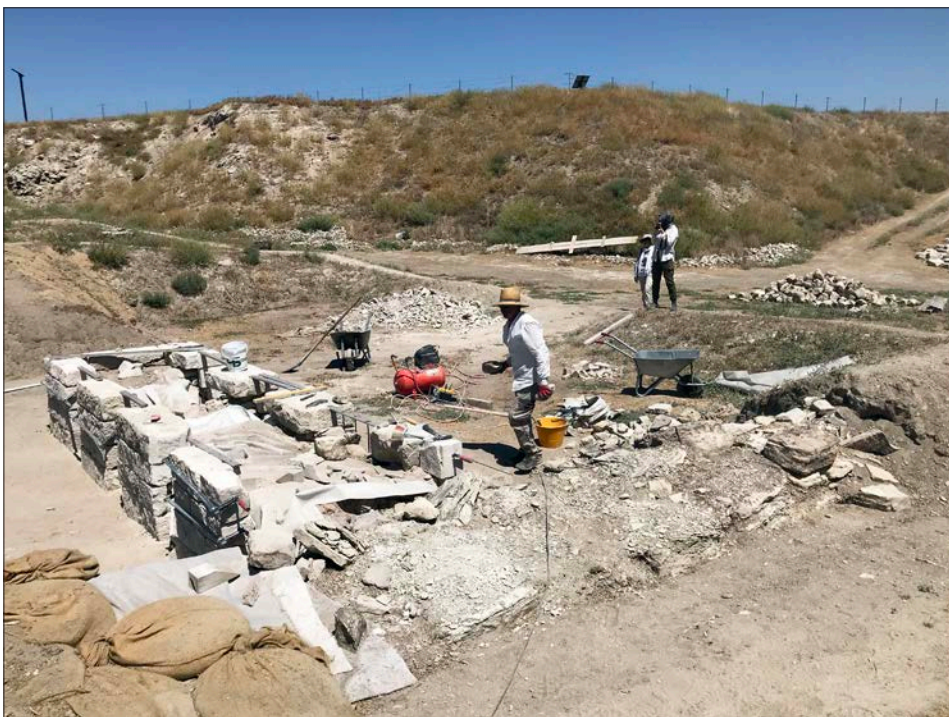
Figure 5: The conservation of Megaron 3, looking west. The disintegrated state of the wall is visible at right; the new stone encasement is at left. Photo by Elisa Del Bono.
